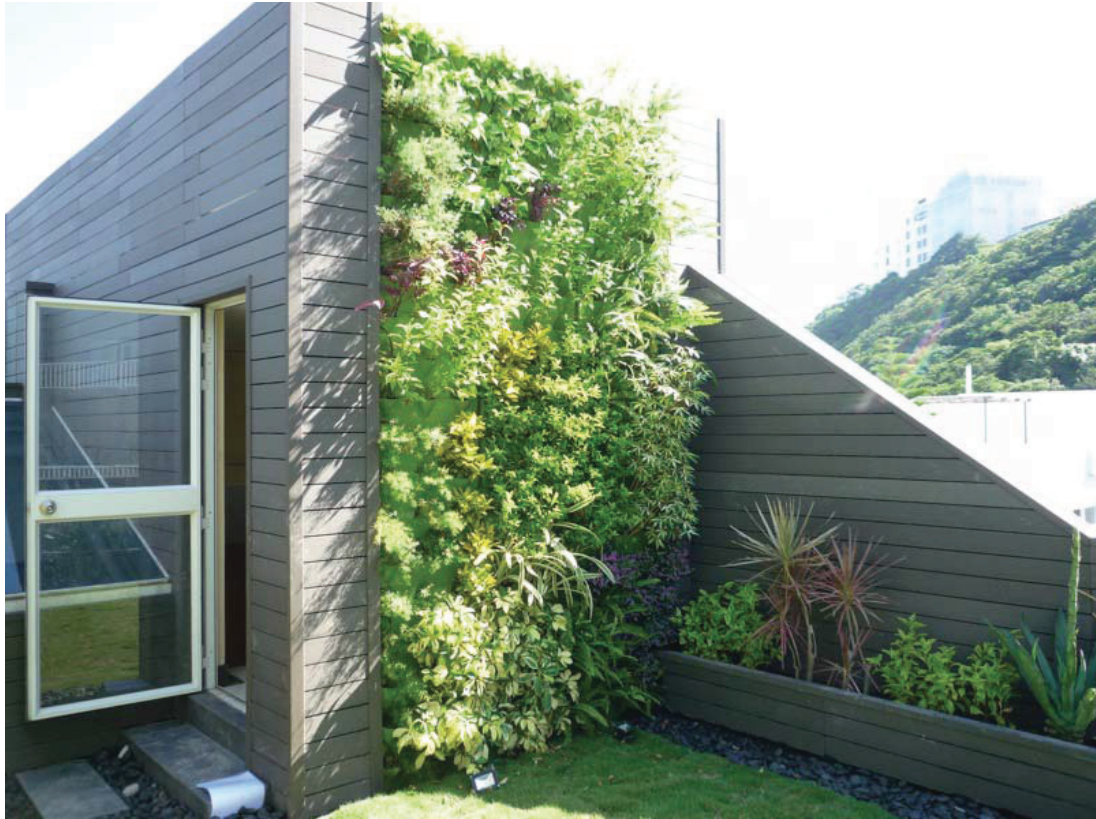
The Peak, Mount Kellett Road Completed in 2011
